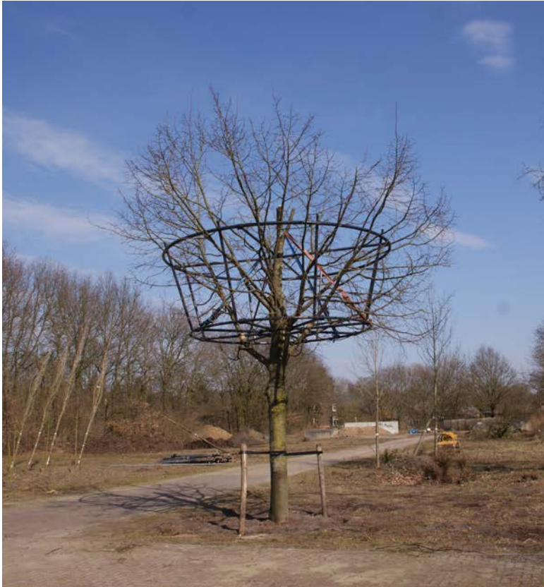
2013 support construction installation and replant
